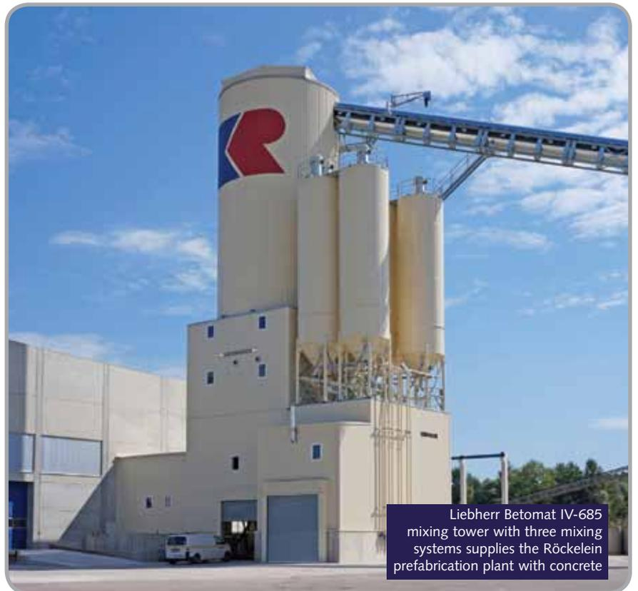
Liebherr Betomat IV-685 mixing tower with three mixing systems supplies the Röcklein prefabrication plant with concrete
